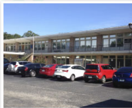
Temporary Main Site, 14 W. Jordan St.
